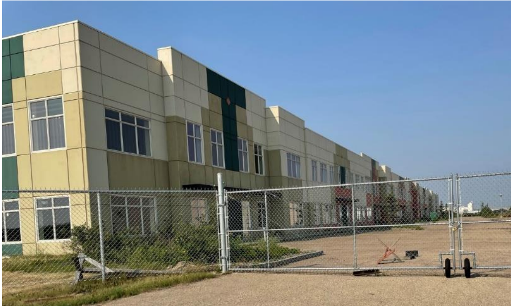
Figure 5: A vacant building on 36 Street
