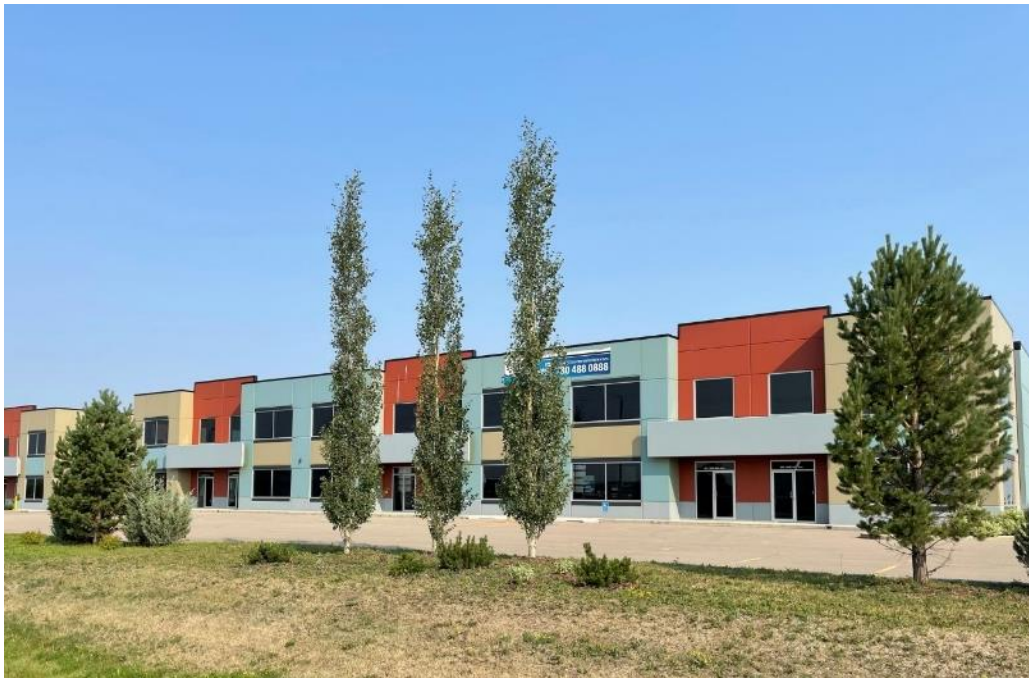
Figure 6: A vacant building on 65A Avenue
