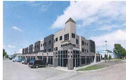
Affordable Housing Gaetz Landing Phase 2
